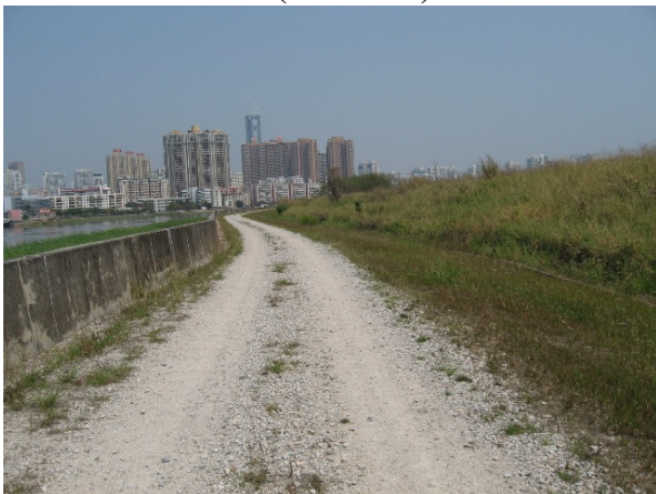
Plate 5 Drainage Maintenance Road located at the north of Lok Ma Chau Loop (Section 2)
