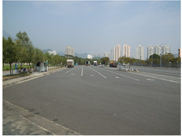
Plate 4 Site of the Boundary Fence to be built in Sha Tau Kok (Section 4)
