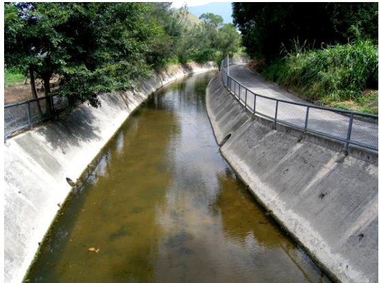
Plate F13 Drainage Channel
