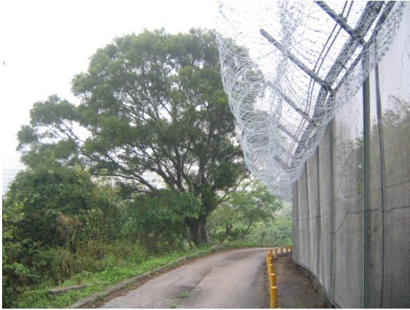
Plate 3 Boundary Fence to be removed in Pak Fu Shan (Section 3)
